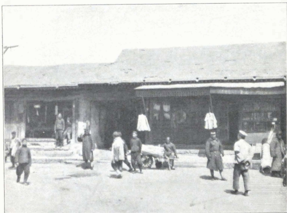
The entrance to our quarters WE ARE DETAINED IN PAOTOW
